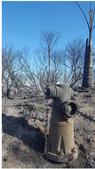
A burnt 2-inch meter (left) and fire hydrant (right) from 2017 Lilac Fire show wildfire's adverse effects on water infrastructure.
