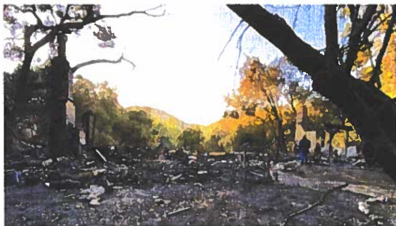
The remains of the Wylie family's home in Fallbrook. Image from GoFundMe page
